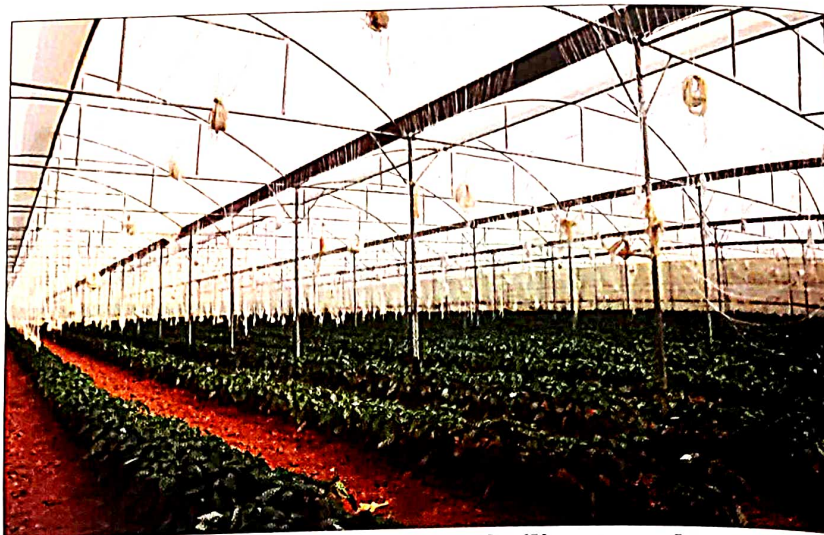
Well constructed polyhouse facilitates good crop
