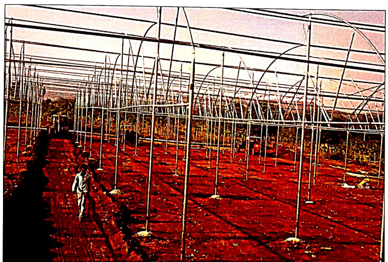
Framework of Polyhouse structure
